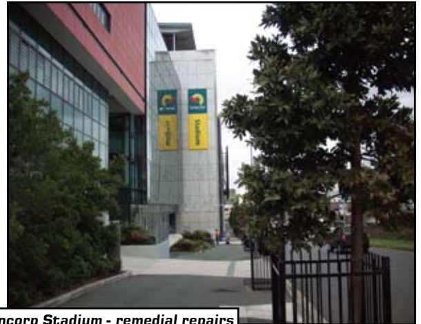
Suncorp Stadium - remedial repairs
