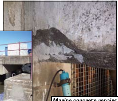
Marine concrete repairs
