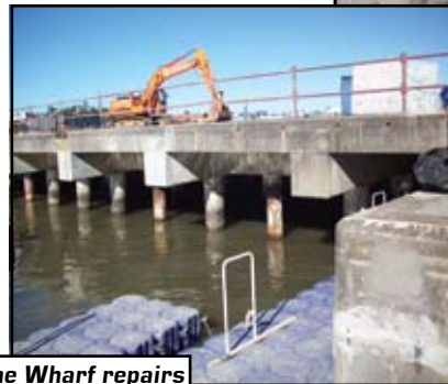
Marine Wharf repairs
